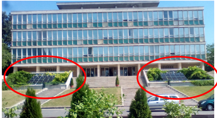
Figure 1. The installed system in front of the Aula building of the campus
